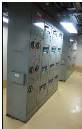
Figure 3: Schematic view of motor control center [12]
